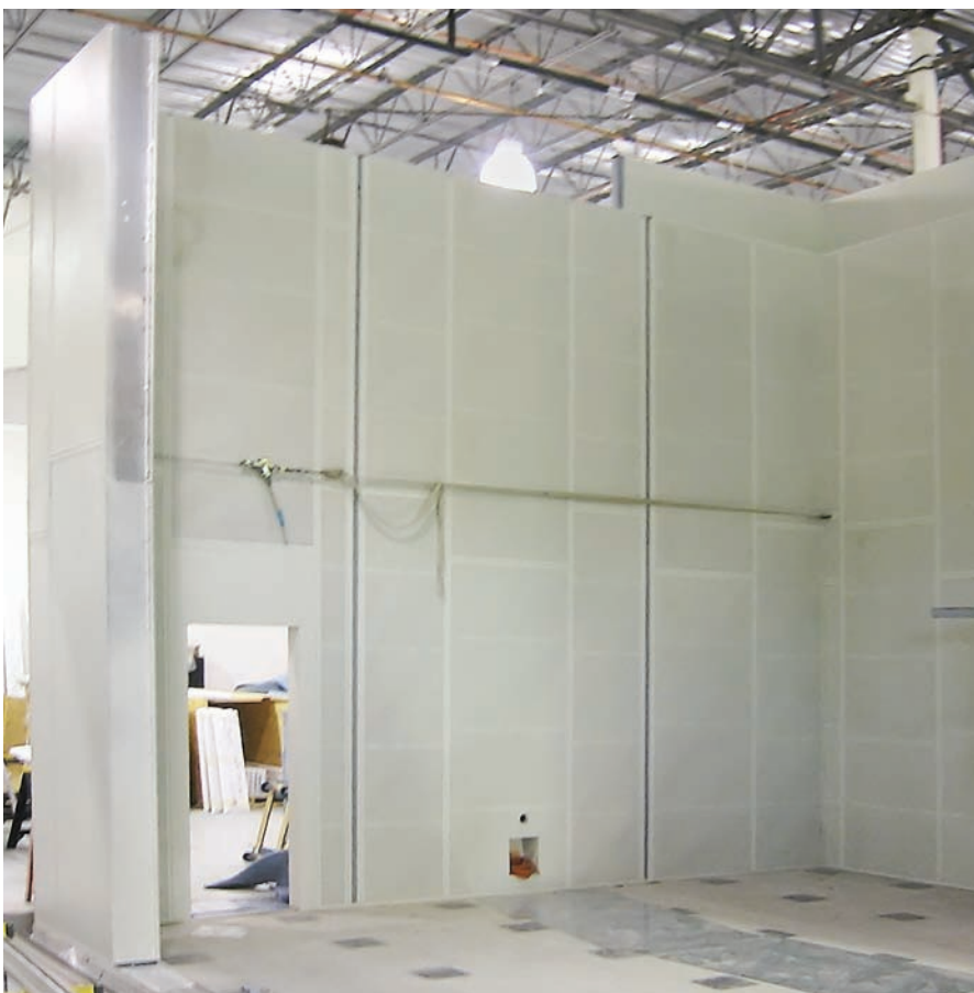
Fig. 5. Inner and outer chamber walls during construction.
