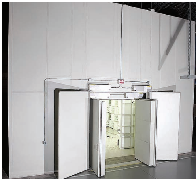
Fig. 8. Completed chamber with double doors open.
