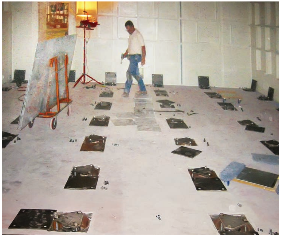
Fig. 3. Raising the inner chamber.
