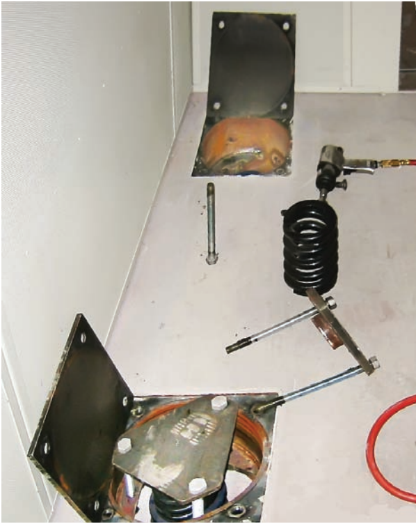
Fig. 2. Spring isolators during installation.
